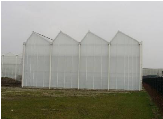
Figure 1: Impression of the 480 m 2 Fresnel greenhouse with 4 roof spans with Fresnel lenses mounted at the south facing roof segments.
