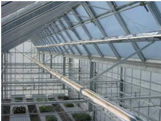
Figure 6: Details of the receivers inside the greenhouse with two receivers per roof
