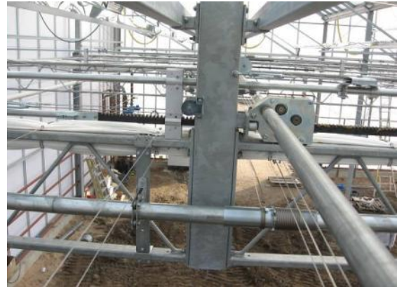
Figure 4: Details of the tracking motor (right) and the gearbox (left) of the tracking mechanism for linear movements.
