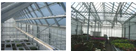
Fig. 2 Details inside the greenhouse Left: The CPV/T module. Right: Overview and cultivation area
