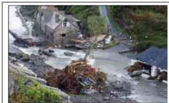
Figure 1. Flood damage caused by high flow velocity (from BBC 2004: http://news.bbc.co.uk/1/hi/in_pictures/3571748.stm ).
