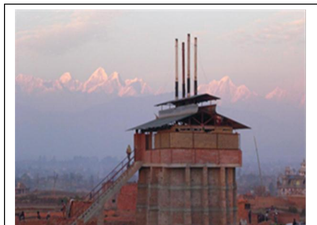
Photo 6.3 Vertical shaft brick kiln (VSBK). (Source: VSBK, 2009).
