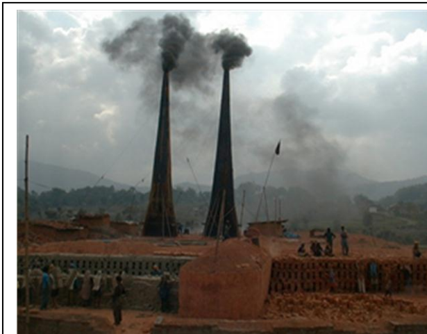
Photo 6.1 Moving chimney bull's trench kiln (MCBTK). (Source: VSBK, 2009).
