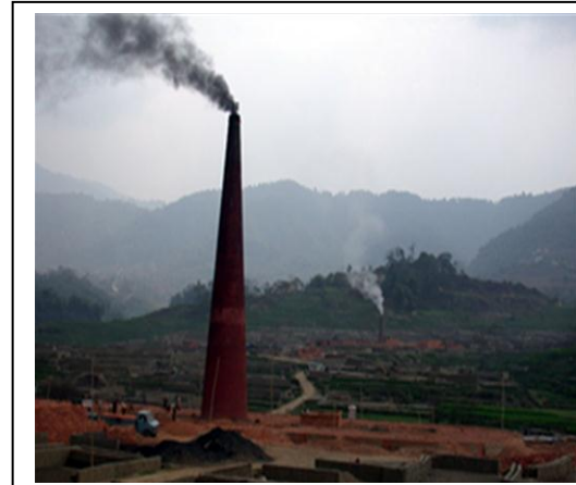
Photo 6.2 Fixed chimney bull's trench kiln (FCBTK). (Source: VSBK, 2009).
