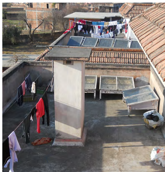
Figure 5.6 Solar panel and solar dryer-panal is used for hot water and dryer is used to dry vegetables to use in winter
