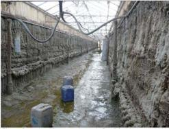
Photo of a pad wall in a greenhouse in Saudi Arabia covered with salt
