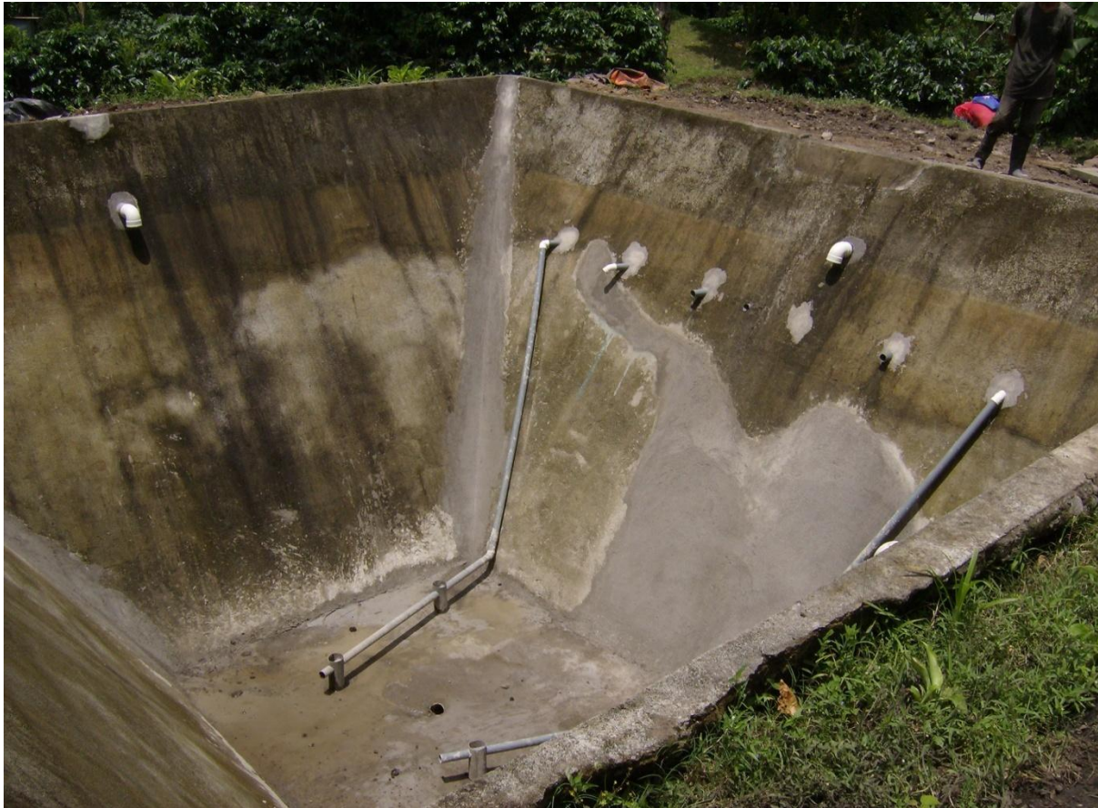
Figure 4: concrete reactor of the LAM system at finca Cueva del Tigre under construction (source: author, 2010)
