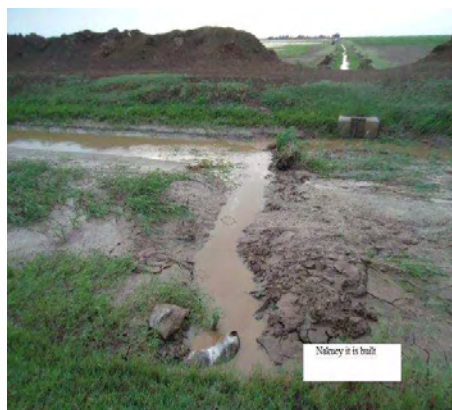
Figure 3.12: farmers create water head with mud on the minor (31-Aug-10)
