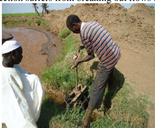
Figure 3.6: Operation of the Tuweir off-take
