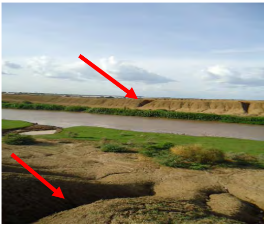
Figure 5.3: Canal banks erosion in the Gezira main canal
