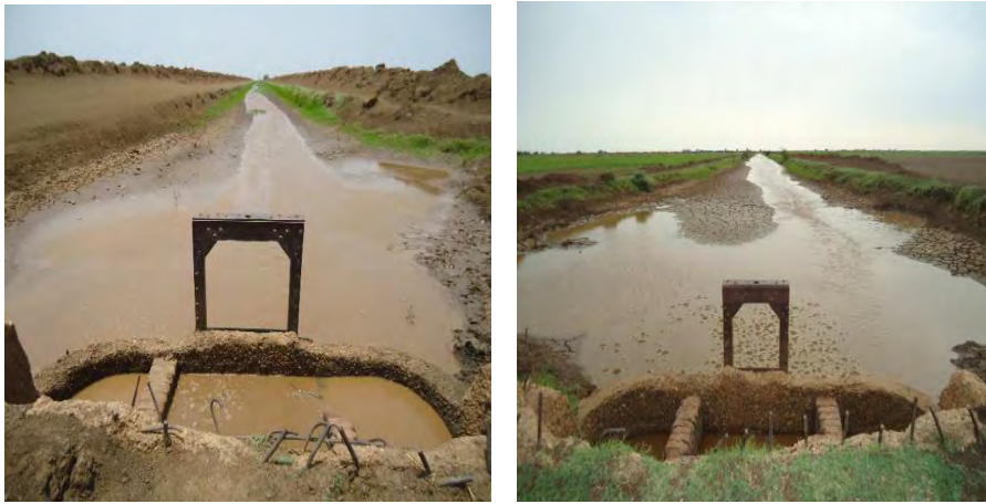
Figure 3.3: Damaged and non-functional NSWs in Tuweir minor
