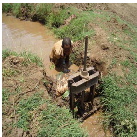
Figure 3.9: A farmer operating a minor off-take Figure 3.10: Pumping from the main Gezira canal
