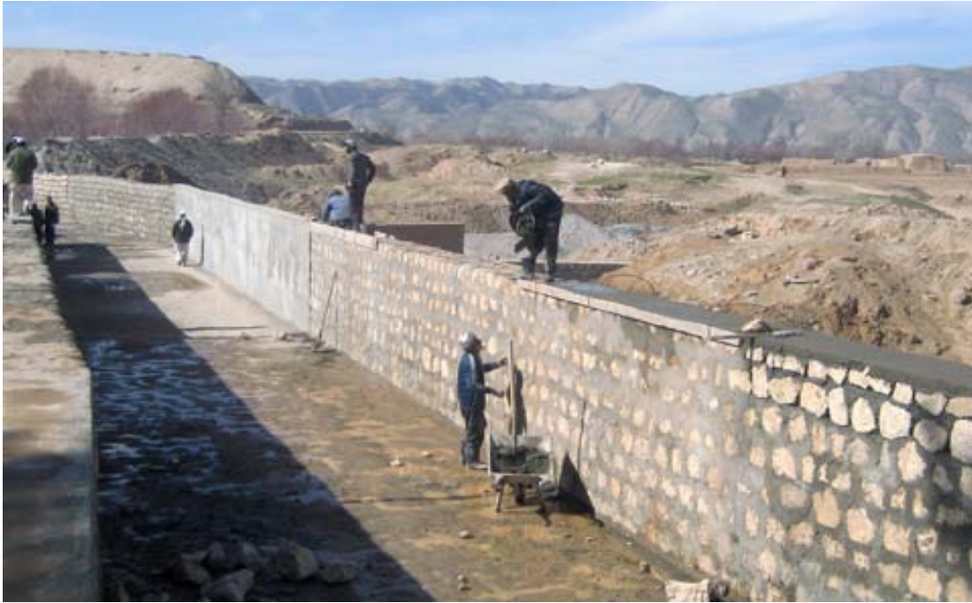
Figure: 3.3: Rehabilitation of Archi canal Source: UNAMA, 2009
