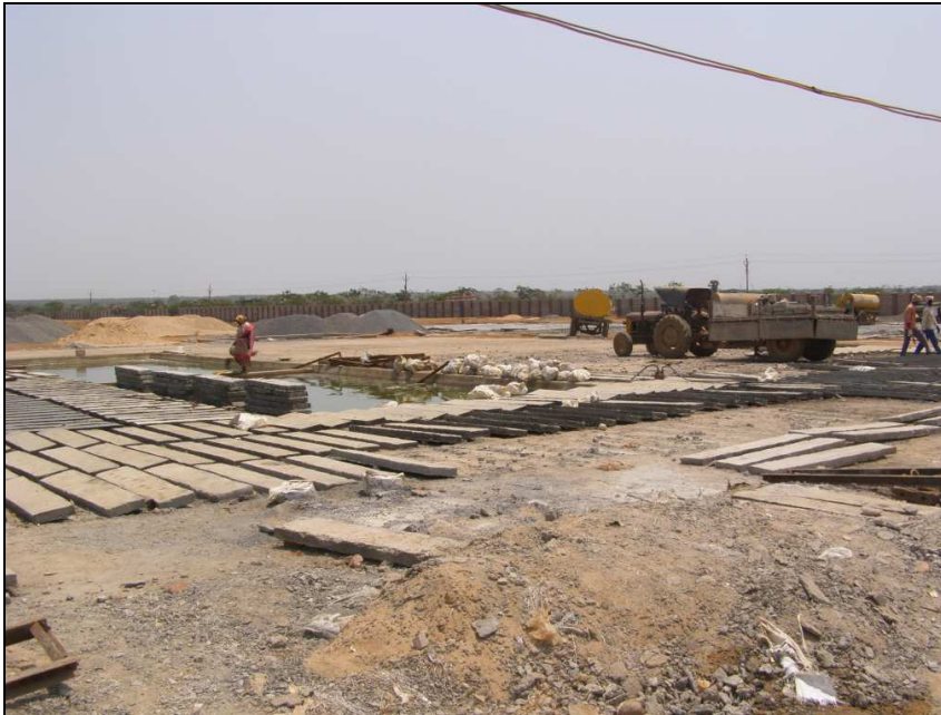
Figure 2.5 Picture of the building of the wall (April 2009)
