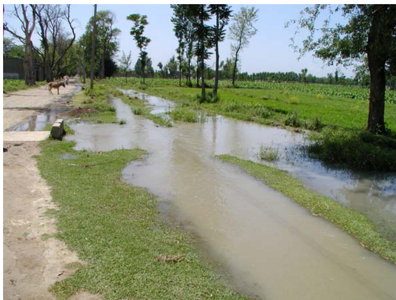
Figure 9.15.A. Flooded tail of a secondary canal due to water refusal upstream
