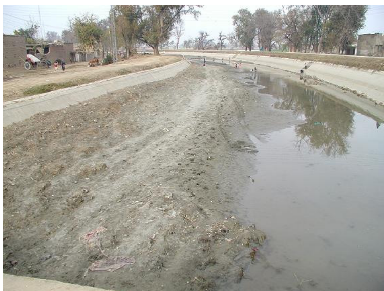
Figure 9.2. Sedimentation in a section of the Lower Machai Branch Canal
