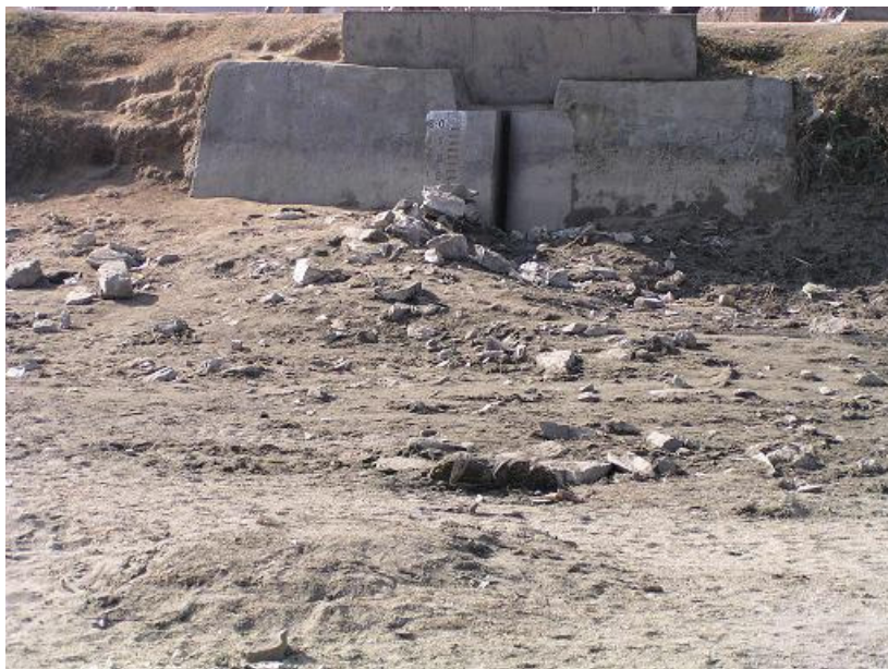
Figure 9.4. Sedimentation in front of an outlet
