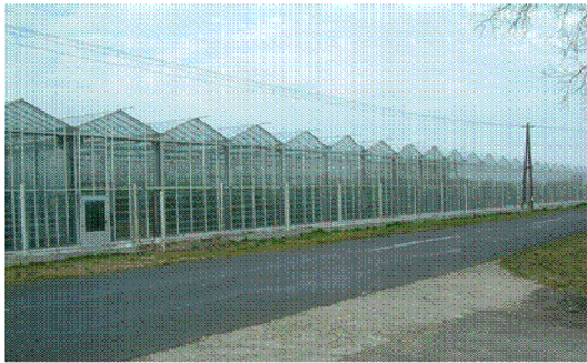
Figure 3.4 Venlo type greenhouse
