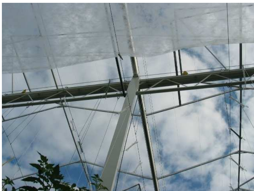
Figure 2.3.2 Venlo greenhouse with steel frame showing inside energy screen
