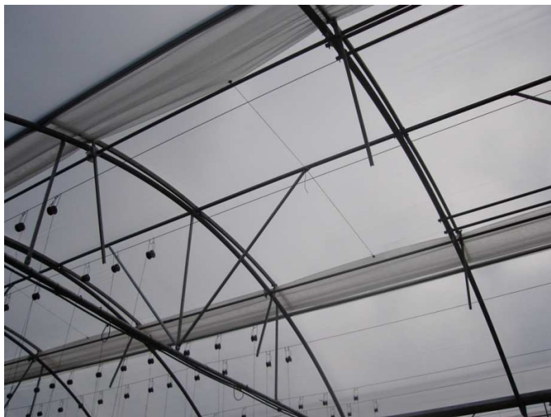
Figure 2.1.2 Multitunnel greenhouse with steel arched roof and plastic covering
