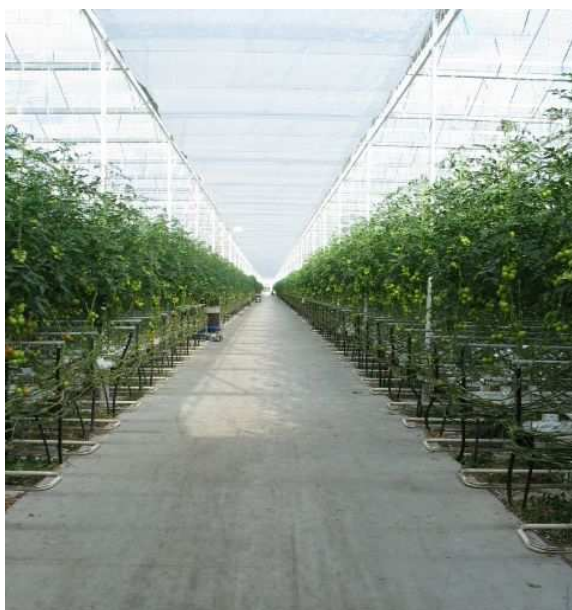
Figure 2.3.4 Heating pipes along tomato rows
