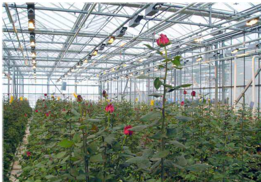
Figure 2.4.2 Lighting installation for rose crop
