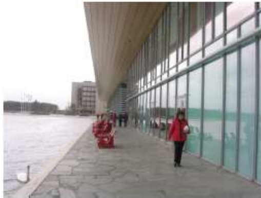
Figuur 3: High Tech Campus Eindhoven (Bron: RJ Fontein)
