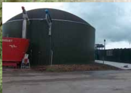
Biogas plant with a feed bunker for dry coproducts
