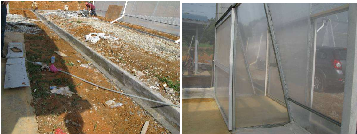
Figure 4. Trash around the greenhouse should be removed (left); the sluice in the greenhouse that must prevent insects from entering (right)
