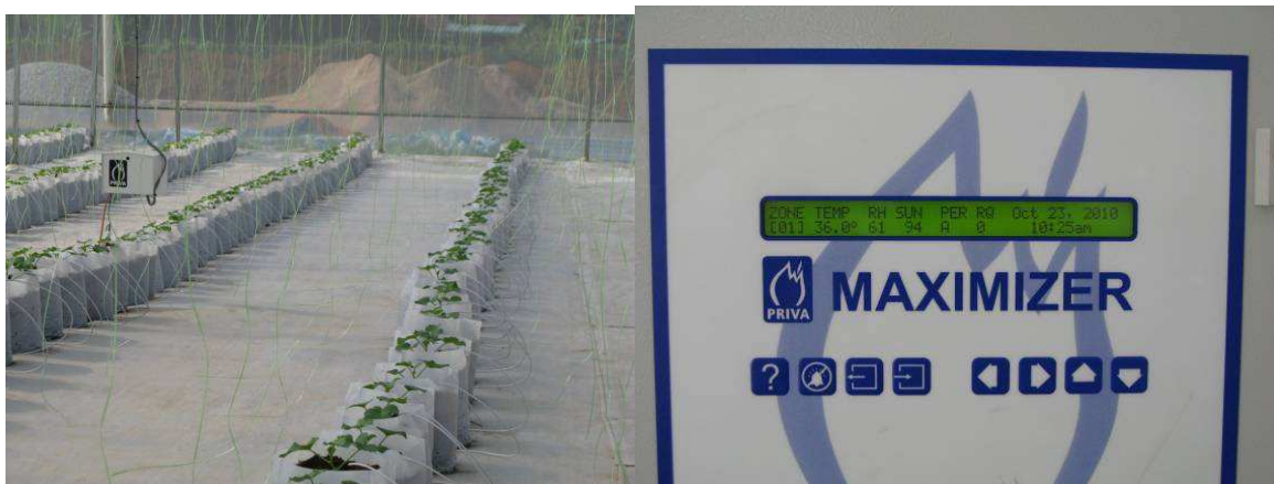
Figure 3. A weather station recording the indoor climate (left); climate data displayed by the greenhouse installation.
