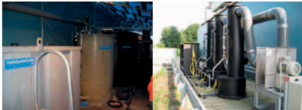
HYDROLYSIS REACTOR AND STRUVITE REACTOR (LEFT) AND STRIPPER UNITS (RIGHT)
