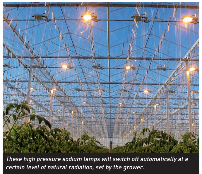
These HPS lamps are mounted under the truss so that they cause minimal light loss due to light interception.
