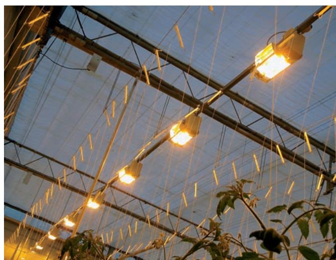
High pressure sodium lamps are the most common type of lamps for greenhouse lighting
