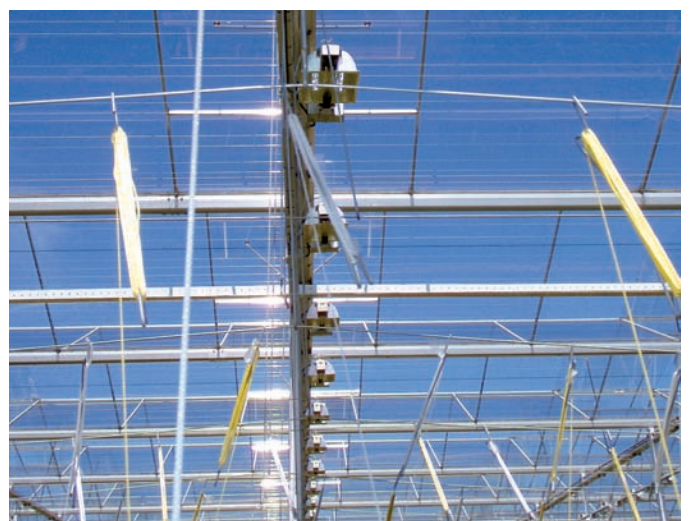
These HPS lamps are mounted under the truss so that they cause minimal light loss due to light interception.
