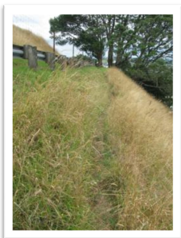
Figure 11 Off side pedestrian track
