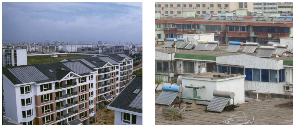
Figure 6.4 SWH installed in apartment buildings (left: integrated in new buildings; right: added to existing buildings)
