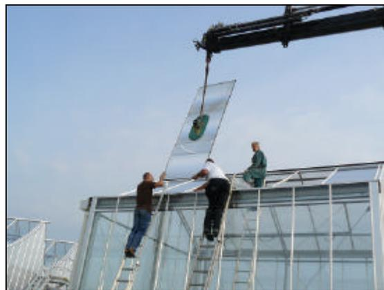
Figure 5 Placement of the Fresnel lenses (placed between double glass).
