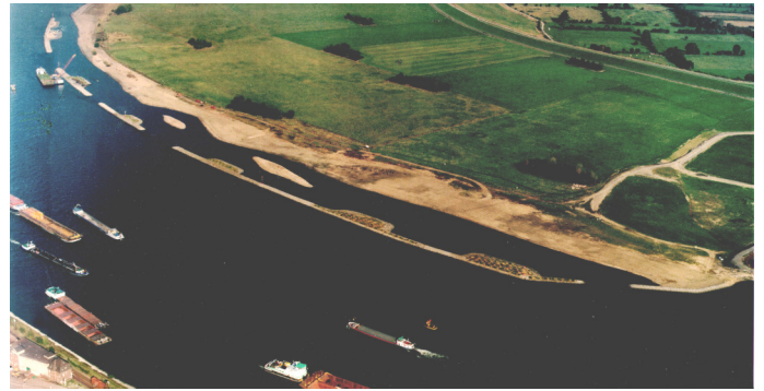
Figure 8: Longitudinal dam in the Rhine river at Walsum-Stapp
