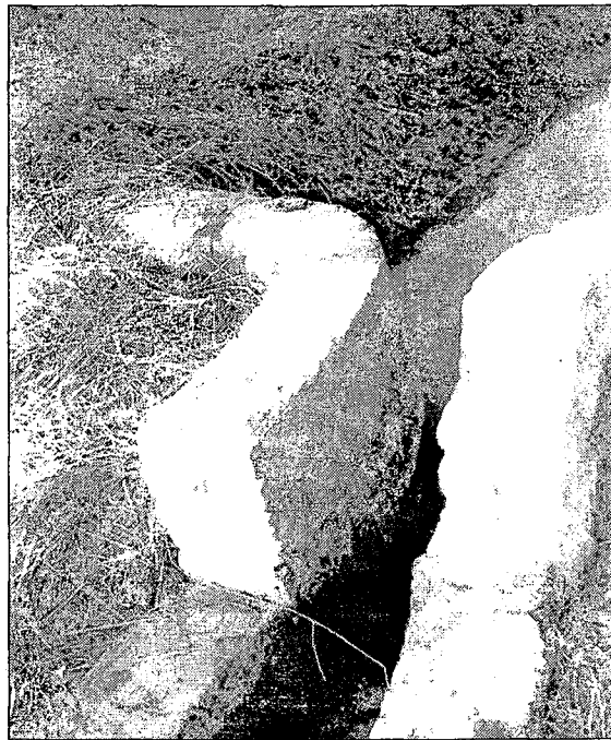
PICTURE 4.4 Open Flume outlet at the tail of the Sitapur Minor
