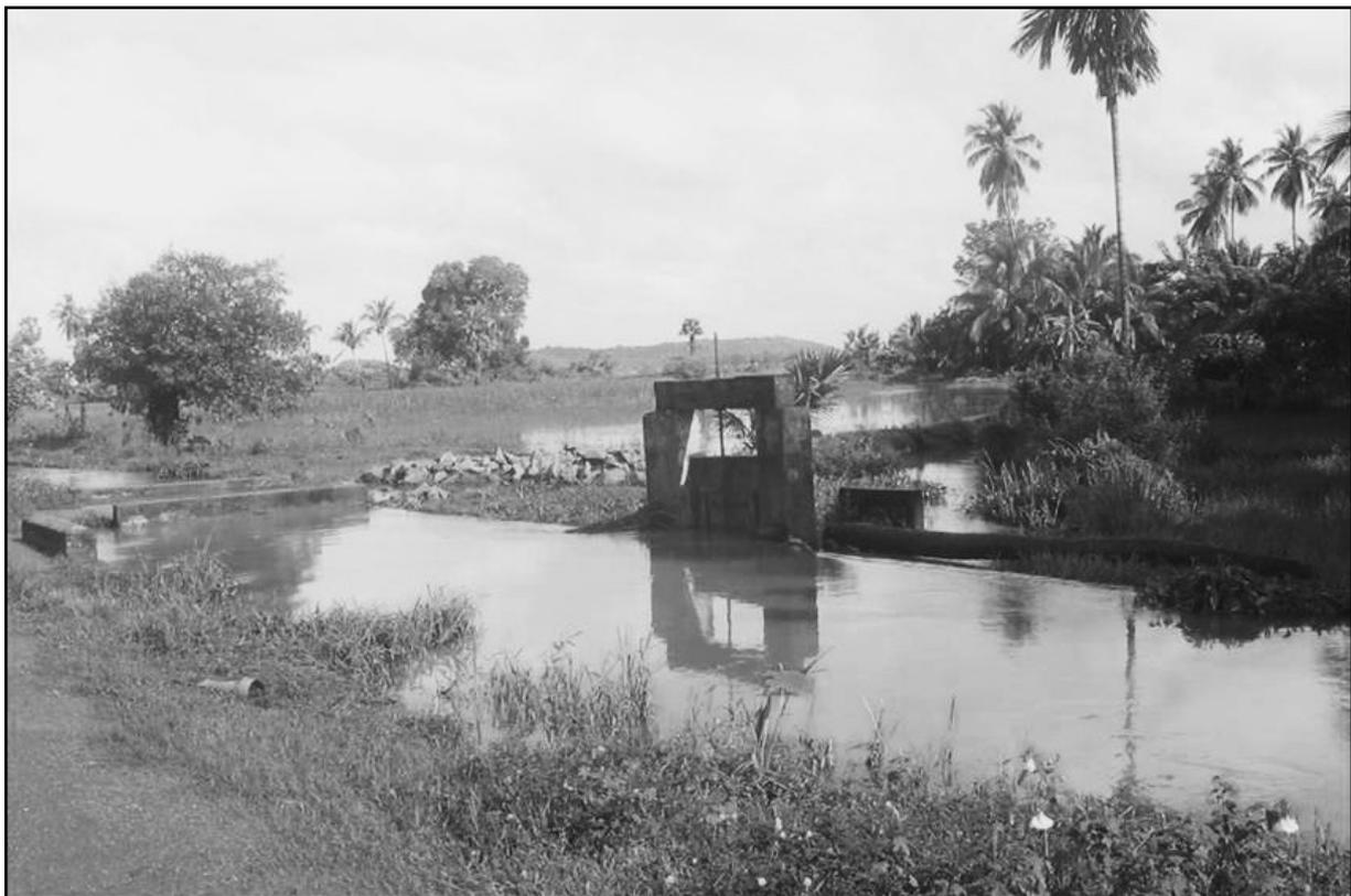
Figure 6.10. Channel filled over maximum capacity (own photograph)
