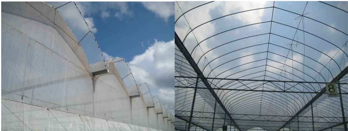
Figure 5. Terengganu greenhouses with gothic roof system and without top opening.
