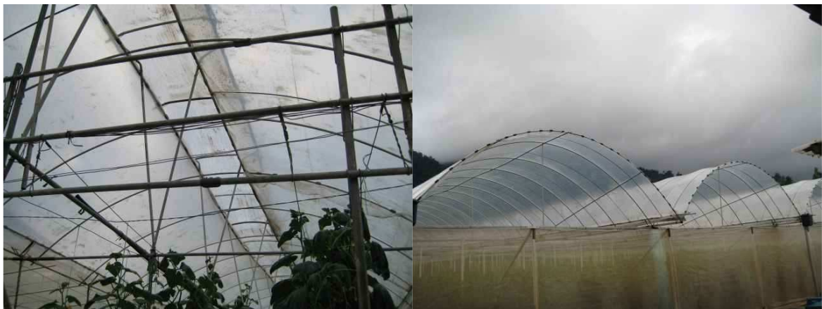
Figure 6. A traditional greenhouse design with a top opening (left), and a traditional greenhouse design without a top opening, as found in most greenhouses in the highlands (right).
