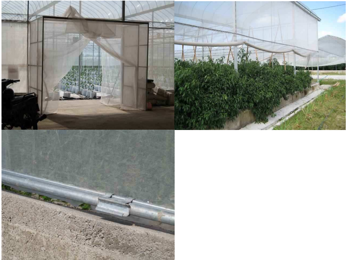
Figure 9. Pest control at TRG Sutratani farm in Ternengganu. Top, left: a greenhouse sluice to limit insect entrance, however not used properly. Top, right: side-walls are not really closed with nets (holes), nets are opened and sluices are not used. Bottom, left: opening in the greenhouse construction that should be closed.
