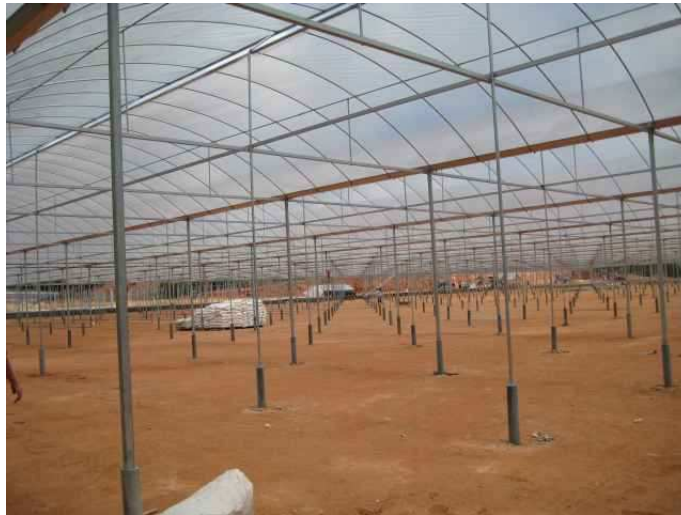
Figure 1. A new greenhouse design with asymetrical (small) roof opening at K.C. Kwan & Sons Sdn. Bhd farm.
