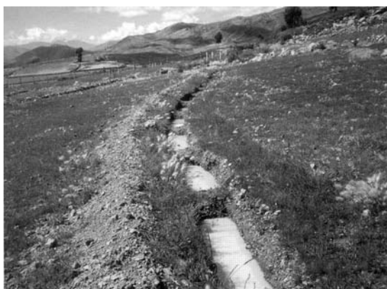
Photo 22: Infiltration ditches
