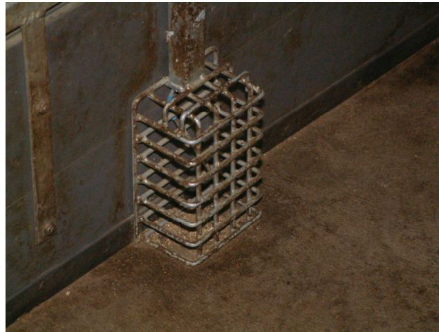
Figure 4. Metal cage to protect AOZ sensors in pens.
