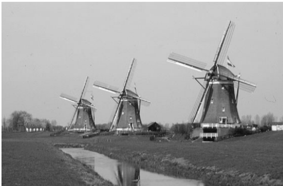
Figure 3.13 Windmills arranged in series of three to pump a polder dry
