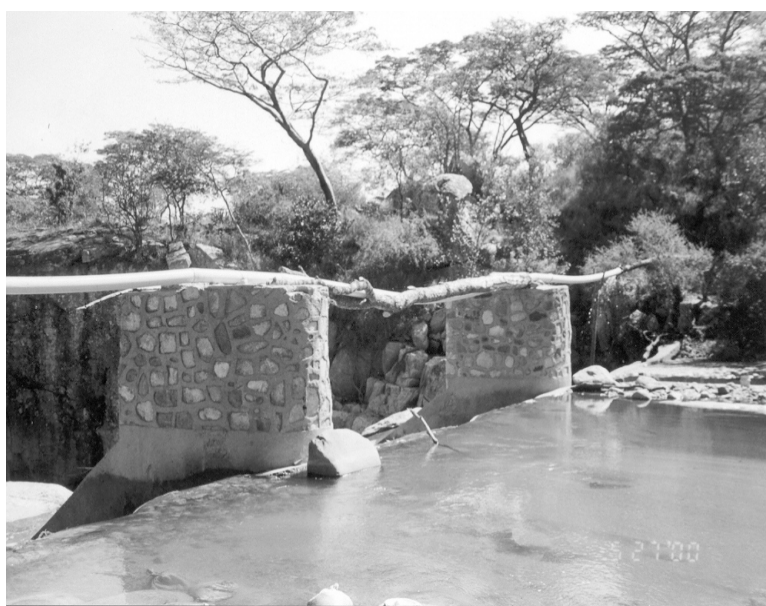
Photo 8.5.2 Farmers' reconstruction upper block -PVC on pillars reinforced with Msasa tree logs against sagging at Mpudzi
