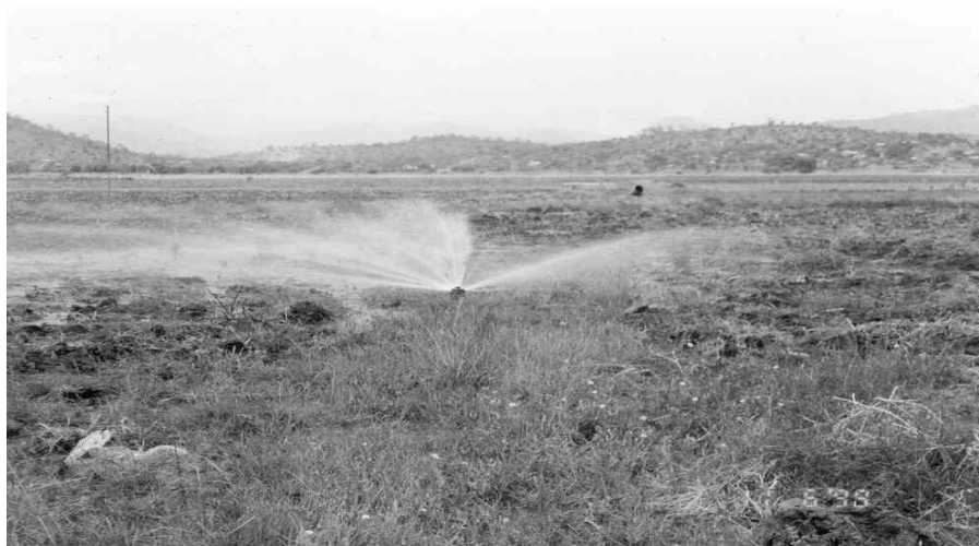
Photo 5.7.1. A typical leaking hydrant in block 11 Mutema
