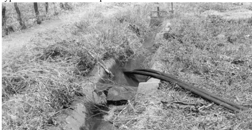
Photo 3.3.4 A typical stone and plastic check at Chakowa
