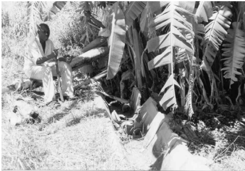
Photo 3.3.5 Bananas undermining lined canal in block A Chakowa
