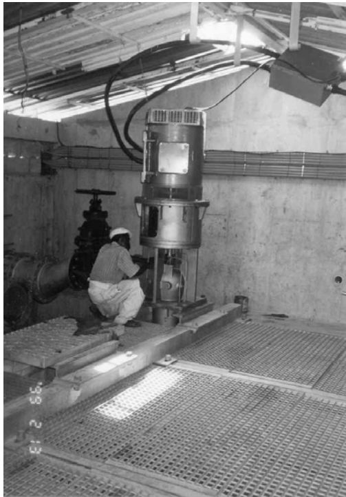
Photo 7.5.2 Vertically mounted motor at Bonde
