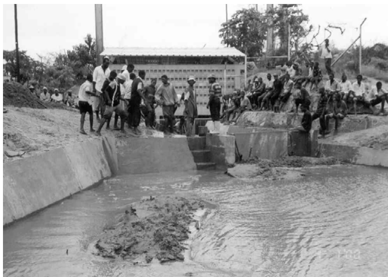
Photo 7.5.1 Farmers desilting the pump intake at Bonde
