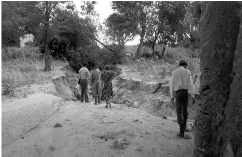
Photo 4.4.1 Main canal breach at Deure in 1998
