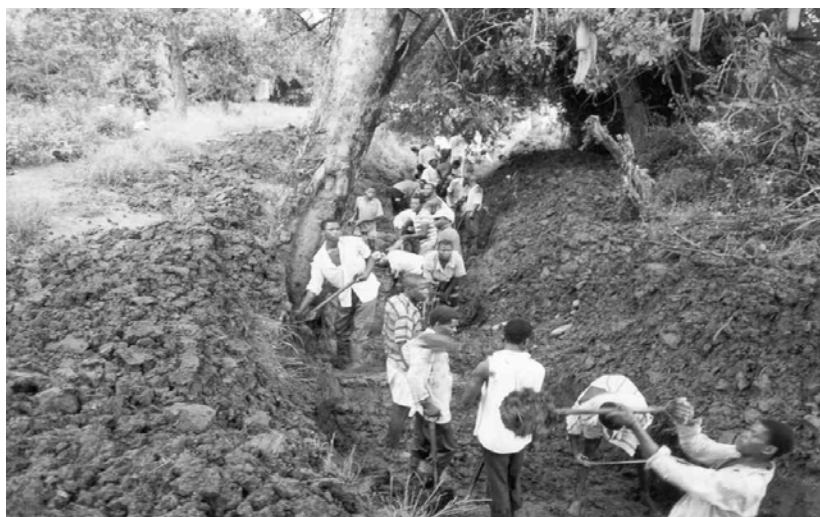
Photo 4.4.3 Desilting conveyance canal after canal breach at Deure
