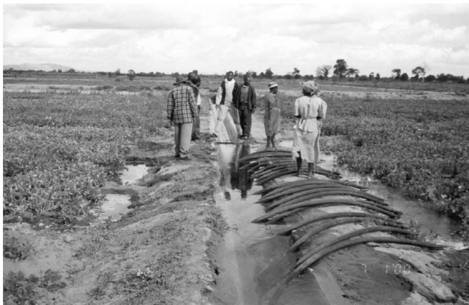
Photo 6.5.1 Siphoning practice on left canal bank and erosion of the left embankment at Musikavanhu
