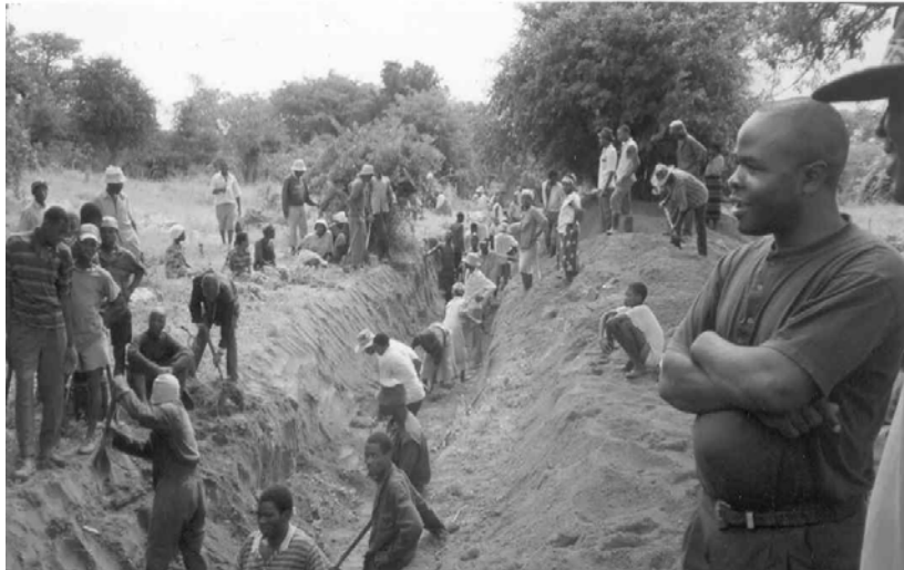
Photo 4.4.2 Farmers realigning canal after breach at Deure
