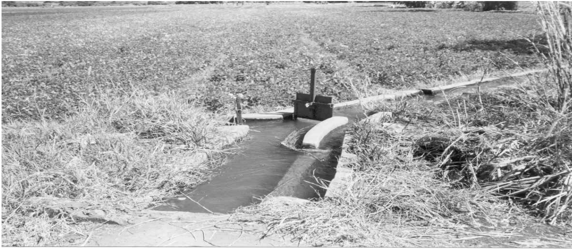
Photo 3.3.2 Gated offtake with internal spillway at Chakowa
