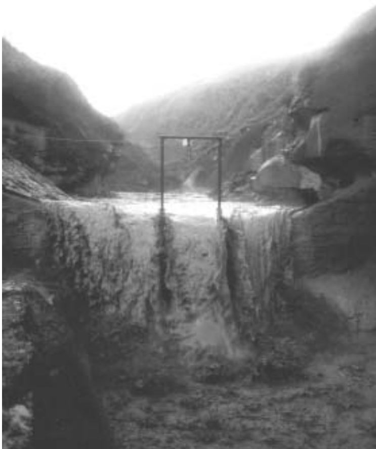
Figure 4.6 Weir at the outlet of the Danangou catchment to measure discharge and sediment concentration. Discharge is measured using an ultra-son sensor, and sediment concentration using an automatic sampler.
