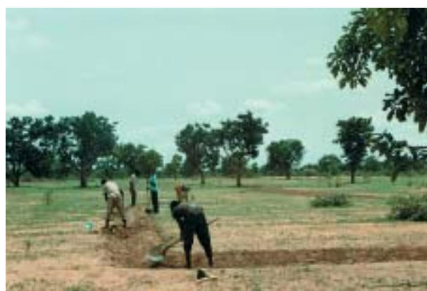
Construction of the 0.5 m high bunds on three sides of the test plot
