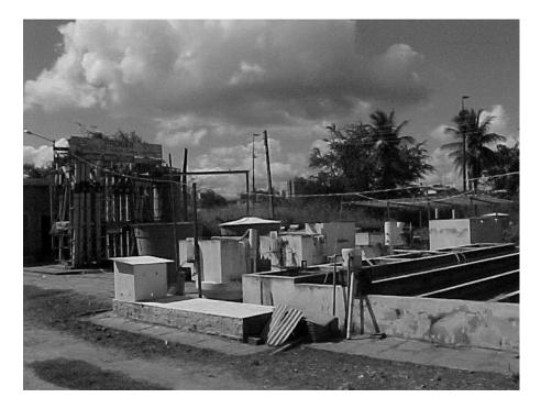
Figure 4.4. Experimental system: UASB reactors and polishing ponds.
