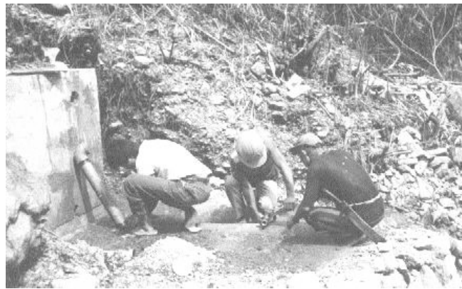
Fig. 1.4 Constructing a water-impounding "spring box."
