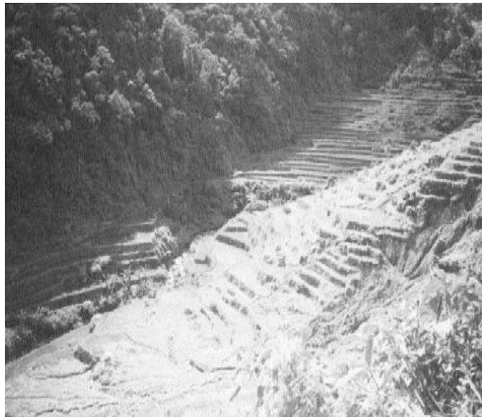
Fig.7.5 Erosion damage on a terrace complex in Bangaan.
