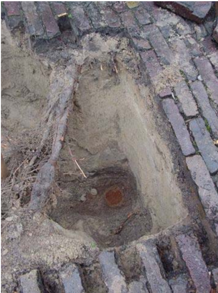
Figure 20 Column of improver Dendromix after removing the overlaying soil
