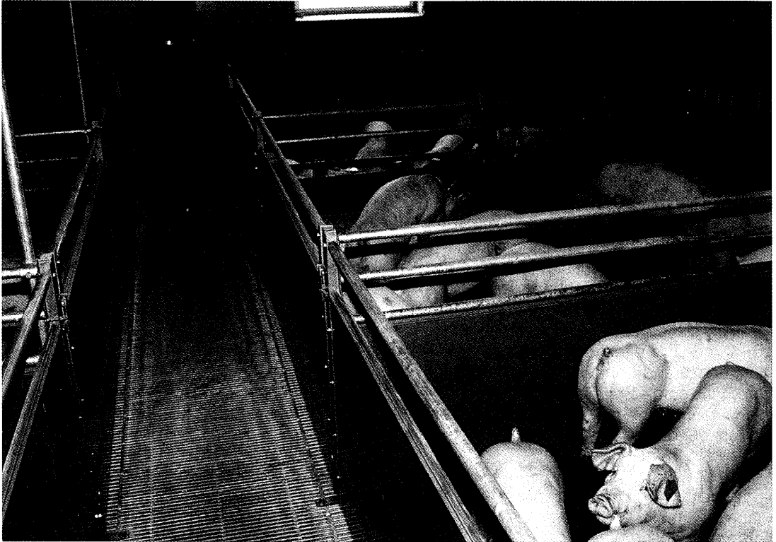
Air inlet via the air channel beneath the feeding alley in the APF facility
