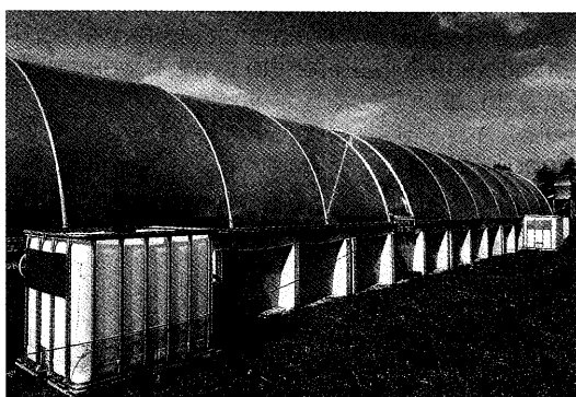
Slurry storage with a transparent foil cover constructed upon a trench silo
