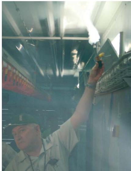
*Controlled side wall inlets allow good air distribution during minimum ventilation.*
