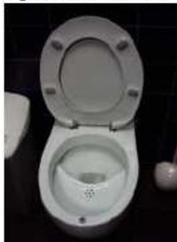
Water use is lower than conventional toilets and as little water is added to the urine to realize concentrated storage. Because of the design of the toilet, men have to sit down when urinating. In Sweden the unwillingness of part of the
