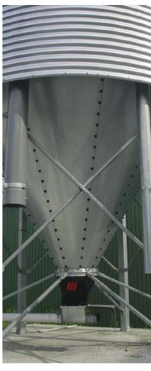
By putting a larger bin over the feed bin the sun has little or no effect on feed temperature.
