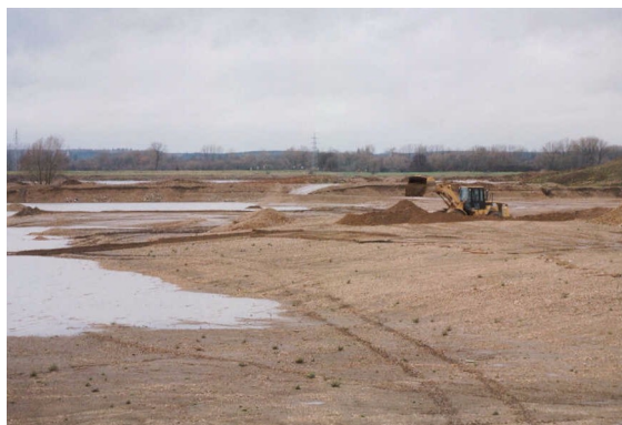
Floodplain lowering along the river Grensmaas, the Netherlands.
