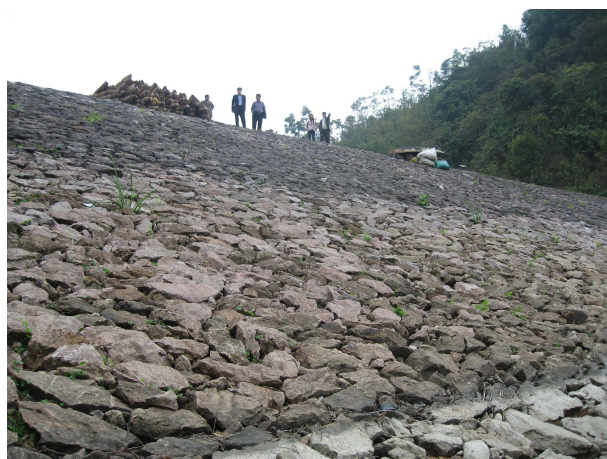
Fig. 4 Upstream slope of the Cap Ke dam
