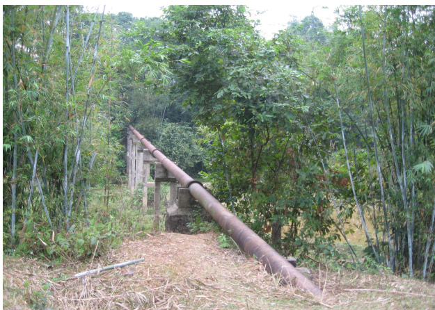
Fig. 9 The Siphon through spring and eroded canal sections
