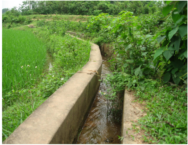
Fig.6 The lined canal in good operation status
