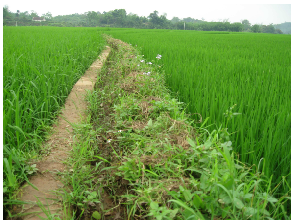
Fig.10 Poor maintenance for secondary canal
