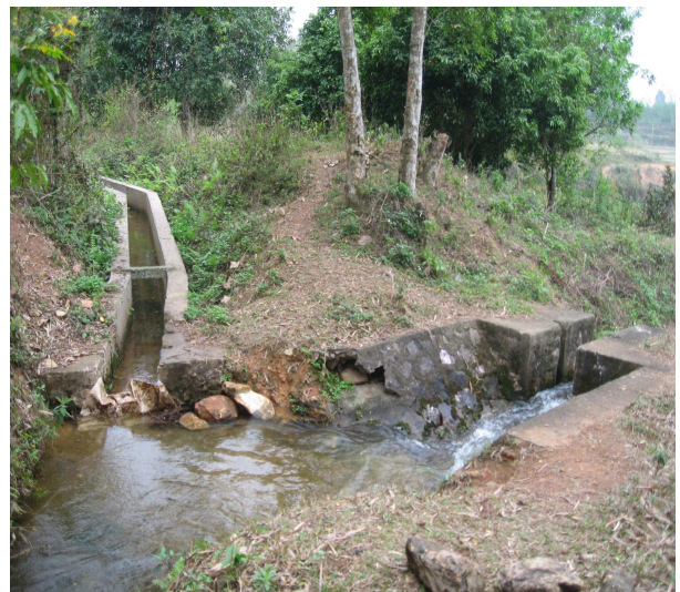
Fig.8 Junction of the Mo sat canal and siphon
