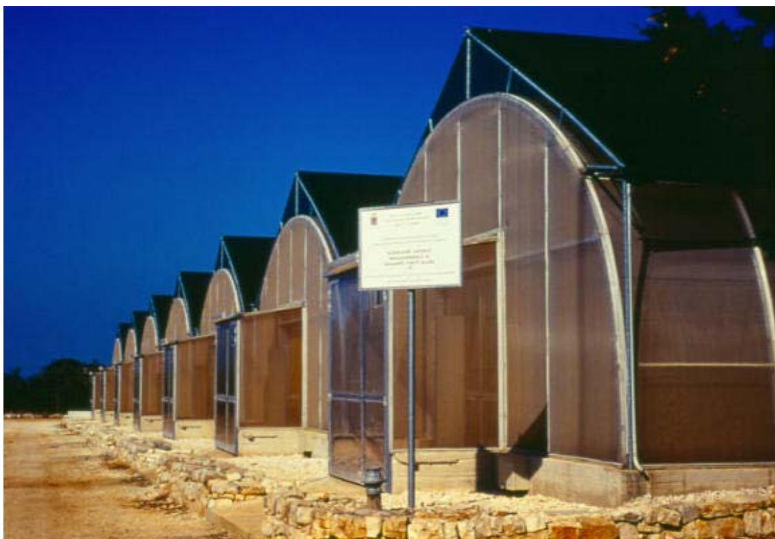
Figure 12. Screen houses for certified crop production with a double layer of anti-insect nets on the arches and with a stand-alone structure for the shading system at the University of Bari (It).
