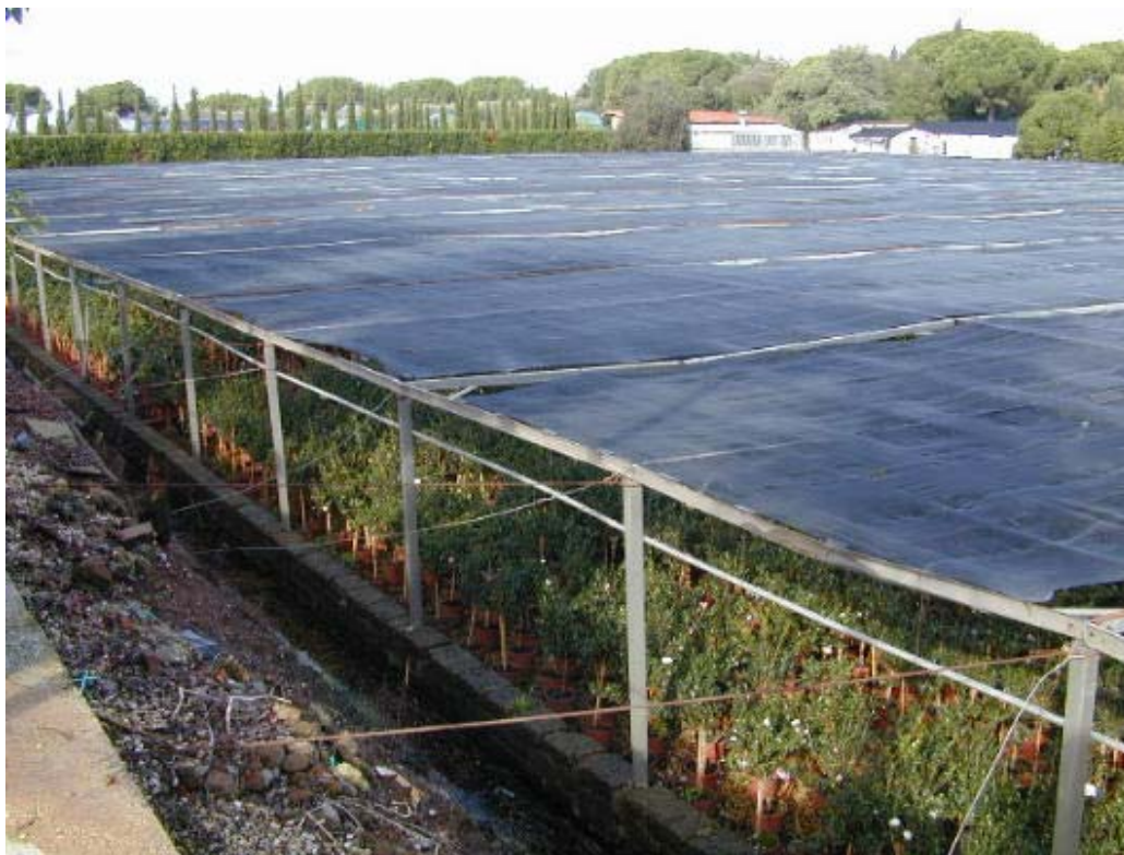
Figure 9. Steel made flat roof shading structure in central Italy.
