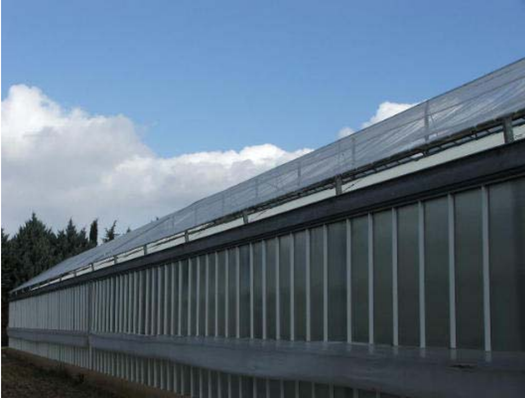
Figure 5. Shading and anti-hail system running over the roof of a glass greenhouse in southern Italy.
