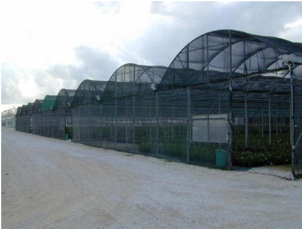
Figure 8. Steel made vaulted roof with eaves shading structure in central Italy.
