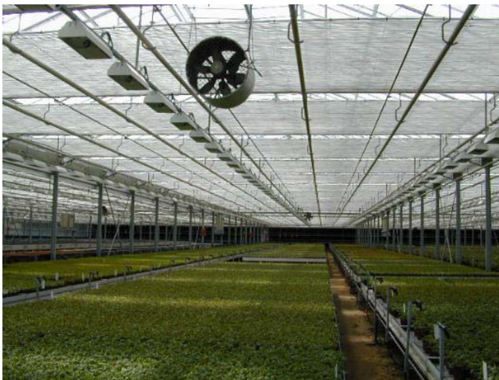
Figure 10. Thermal and shading screens inside a greenhouse in northern Europe.
