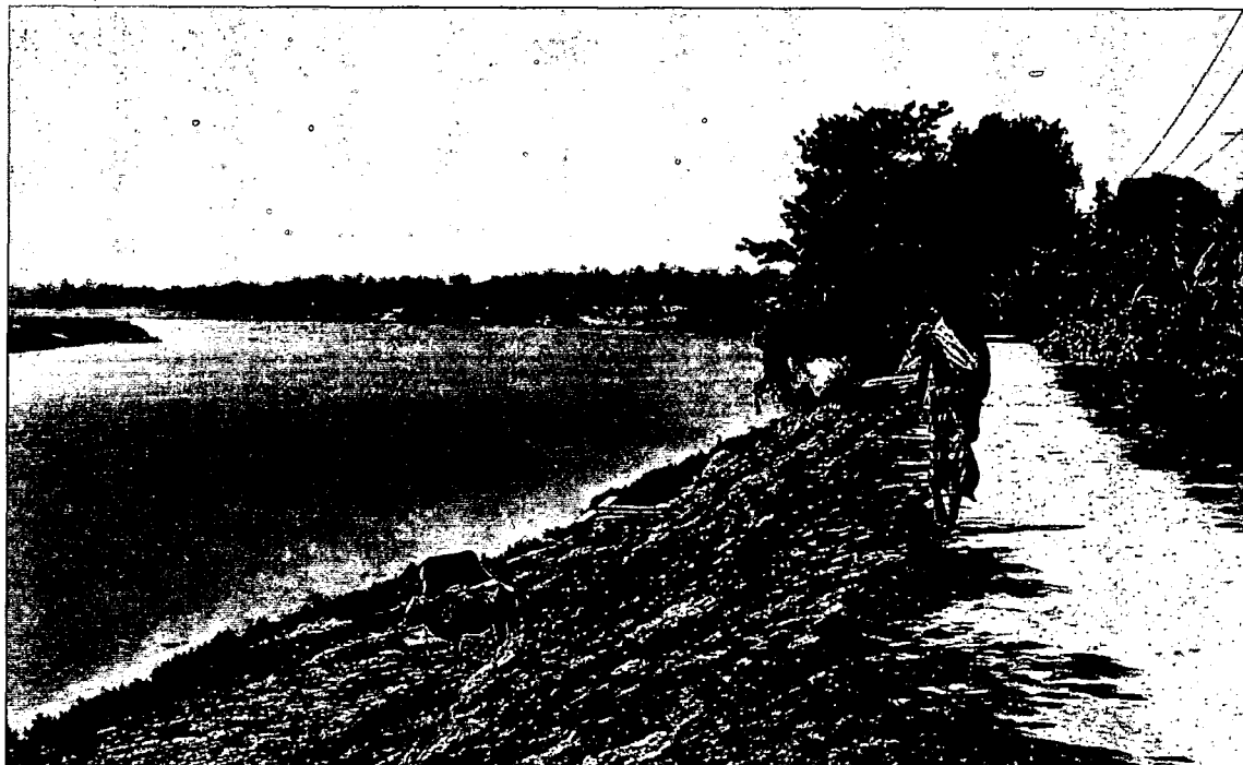
Photo 1 A flood protection embankment
