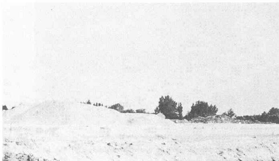
Photo 1. Nederhorst den Berg. The large hillocks of sand that are to be seen, are meant as extra raisings to speed up the settlements on those spots where the total settlements will be largest
