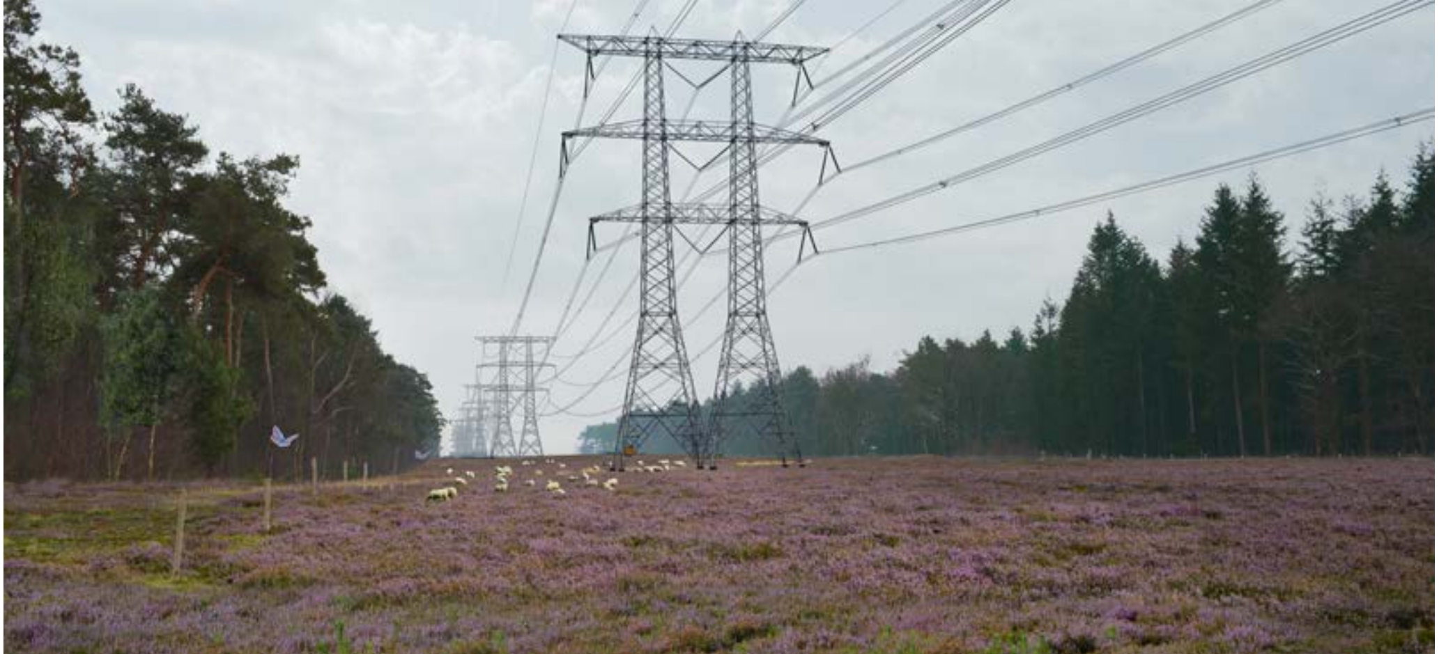
fig 6.21: Power line through the heather landscape
