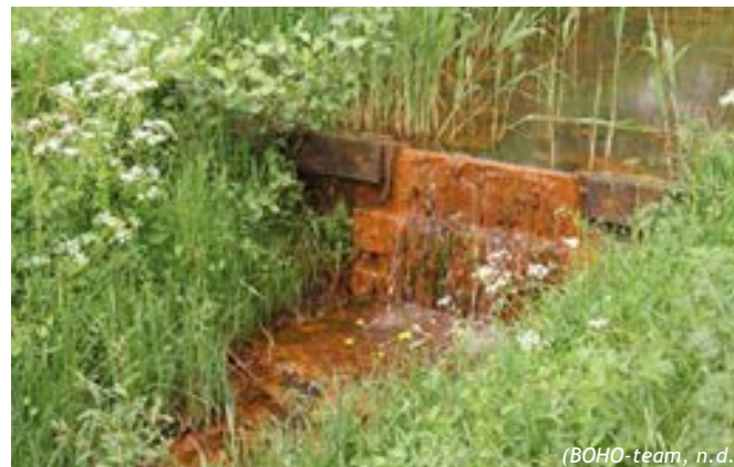
fig 3.23: Oxidating seepage water from the Peelrand crack
