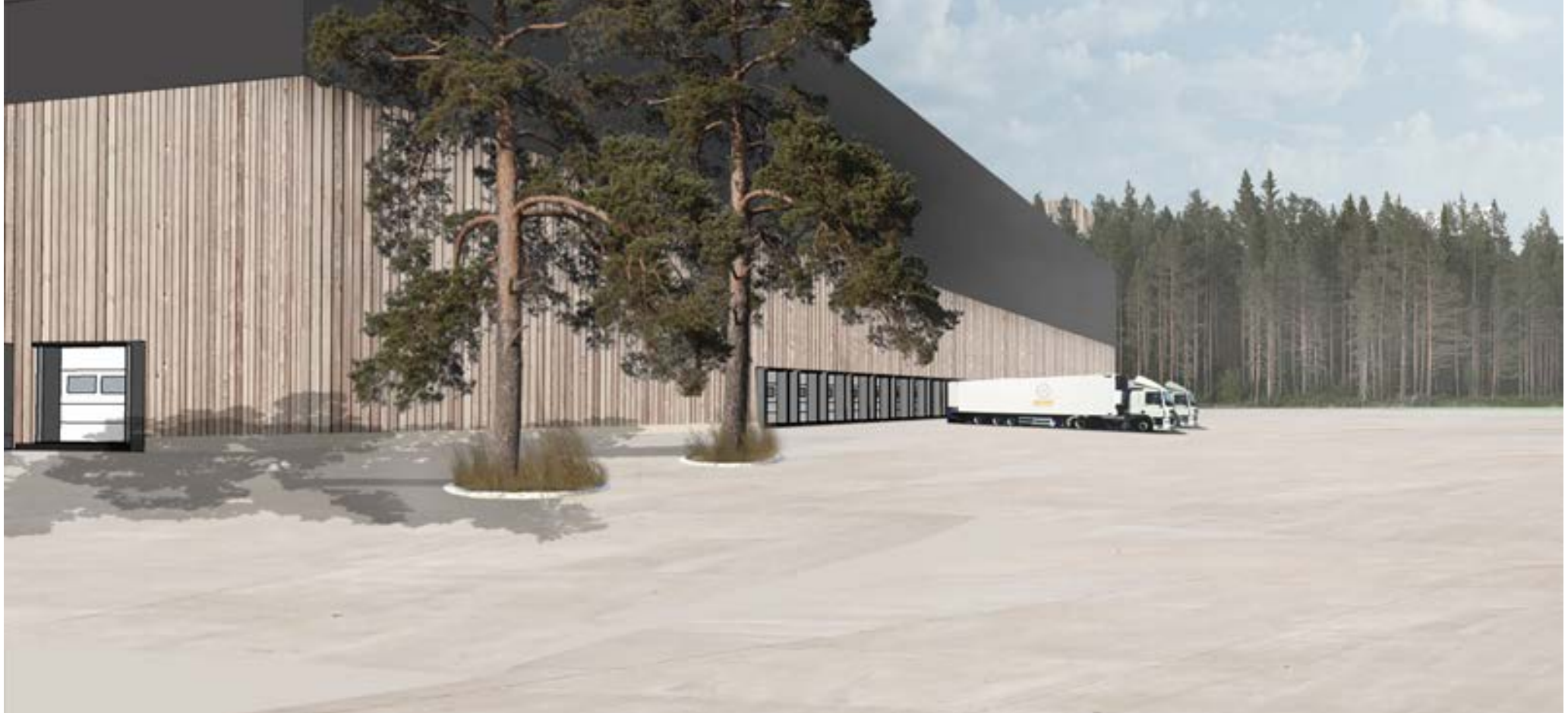
fig 6.25: High bay logistic hub
