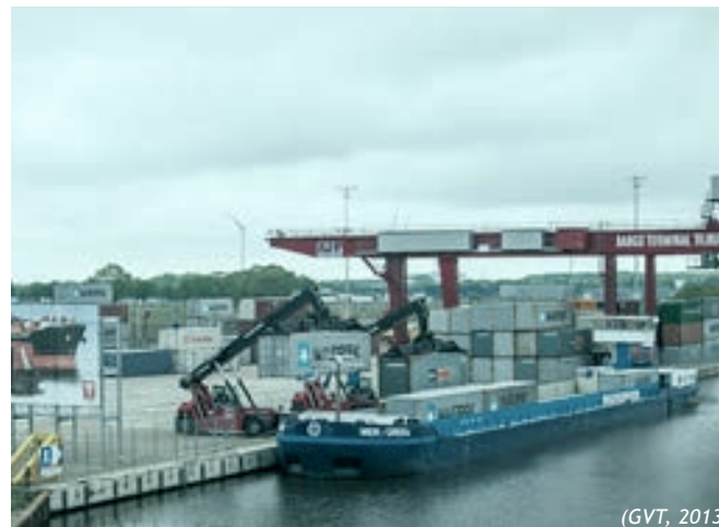
fig 2.35: Inland Terminal Tilburg
