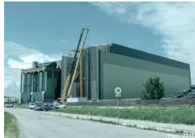
fig 2.21: High bay warehouse (Vipa, 2018)
