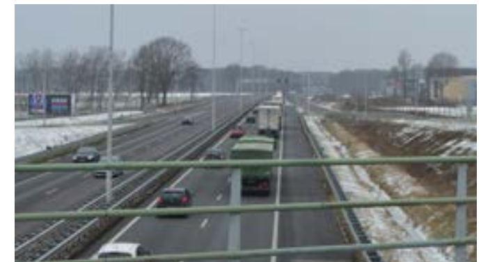
fig 5.21: A58 highway at Moergestel junction
