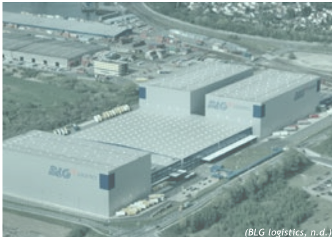
fig 2.23: Large high bay warehouse, Bremen
