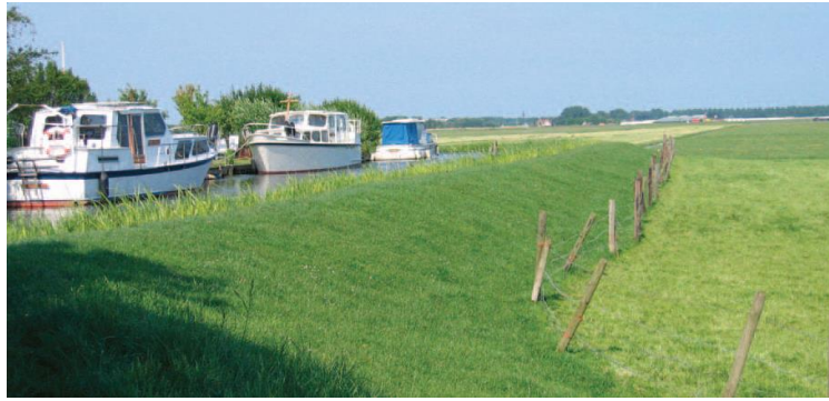
Figure 4-3. Example of canals in Rijnland, where the water level is higher than the surrounding fields
