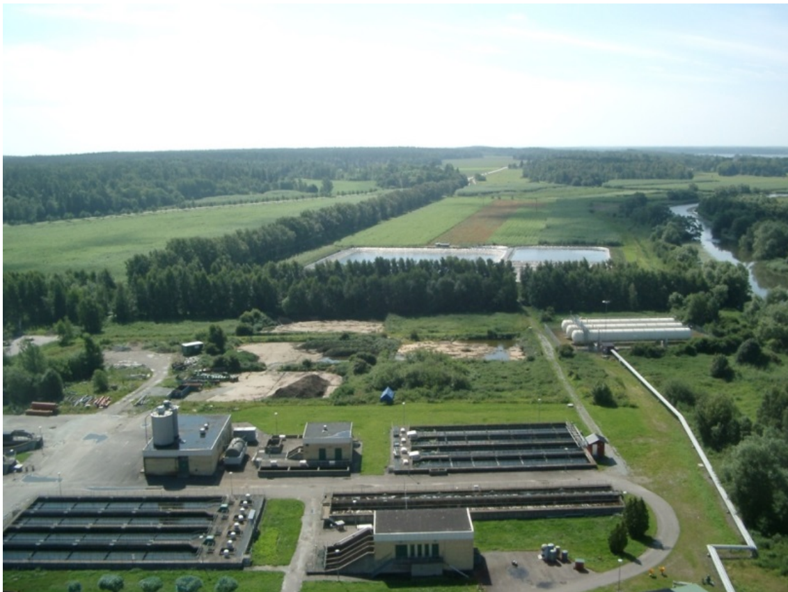
Figure 14: (Case 6) View of a municipal wastewater plant in Enköping, Sweden, with water storage ponds and (behind the ponds) willow fields that are used as vegetation filters. The photo is taken from the roof of the heat and power plant that uses the locally produced biomass (Photo: Pär Aronsson, SLU).
