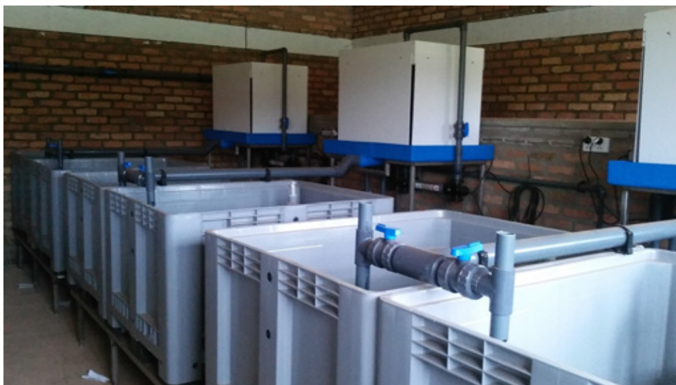
Photo 2 Recirculating Aquaculture System for breeding of Catfish, Huye, Southern Province
