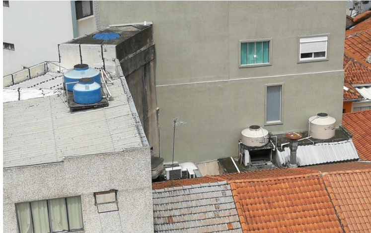
Water storage tanks (caixa da água) on top of apartment buildings and houses in Vila Clementino, São Paulo (2018).
