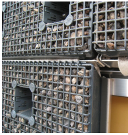
Figure 10 | Gravel filled gabions by Optigrün (Optigrün, 2015)
