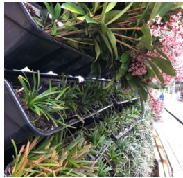
Figure 13 | Planter box system by Gsky (photo by Klapwijk, 2018)
