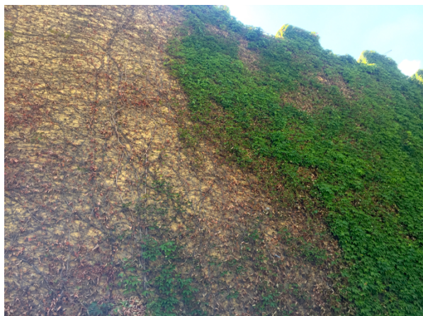
Figure 24 | Failing creepers (photo by author, 2018)
