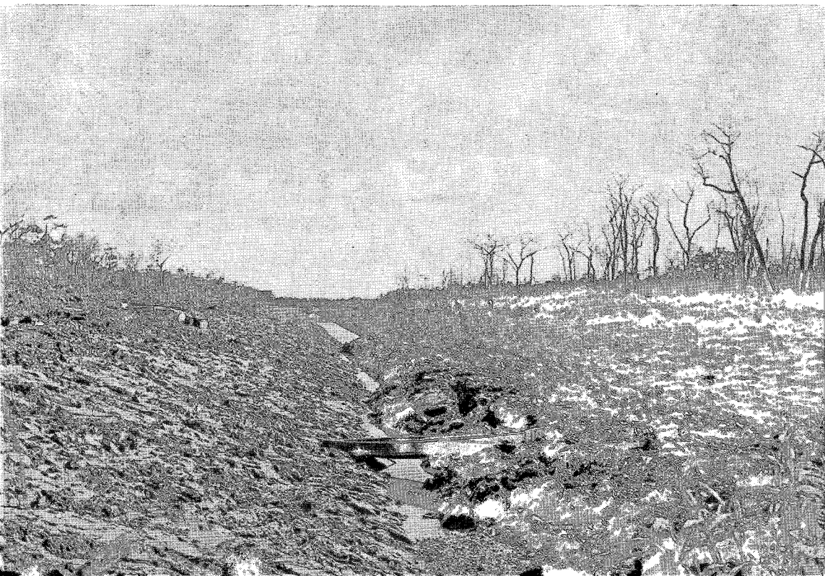
4. Subsidence of talus in main drainage canal, shortly after excavation.
