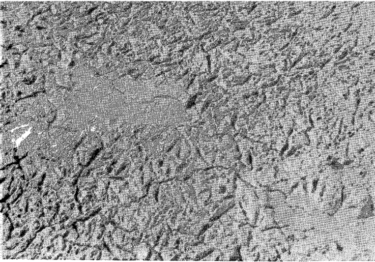
48. Footmarks of ducks indicate cause of damage.
