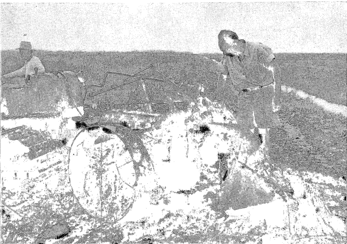
17. Ransomes Solotrac plough with International disk-coulter: although the plough has ample clearance it still is subject to trash clogging and winding.
