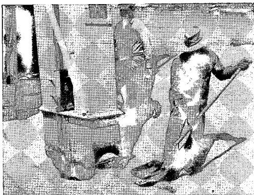
62. Unloading the lighters by scoop elevator at the processing plant.
