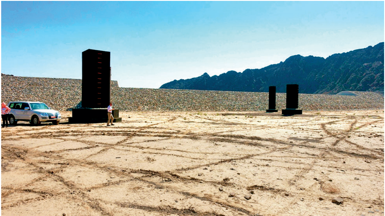
Recharge dam, also for mitigating floods. Black pillars protect shafts of falaj system of flooding
